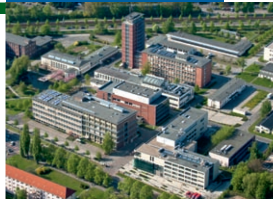
UFZ offices in Leipzig, Permoserstrasse 15
