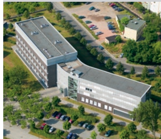
UFZ offices in Magdeburg, Brueckstrasse 3a
